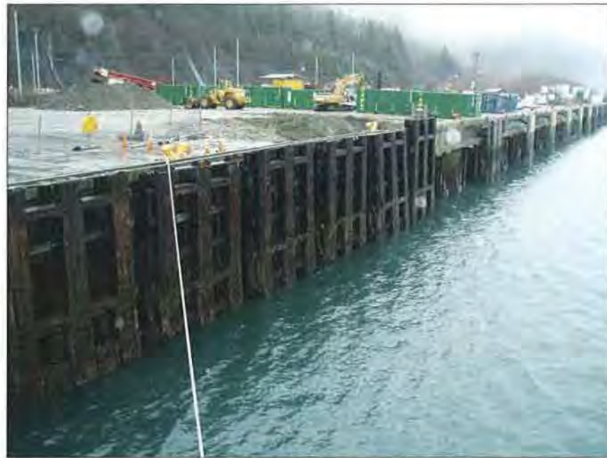
2 38 LUTAK DOCK - DOCK FACE
