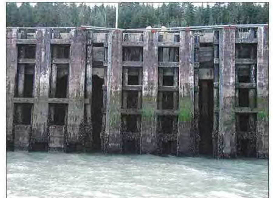
4 38 TYPICAL FENDER MODULE
