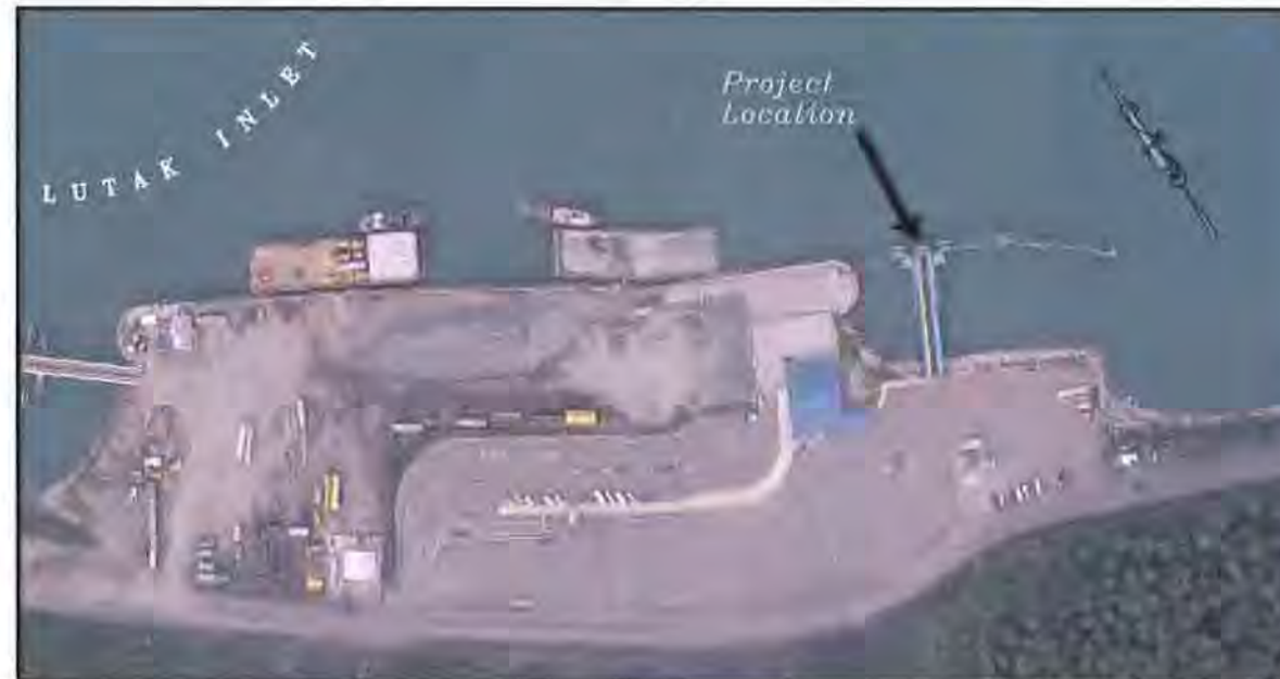
EXISTING TERMINAL SITE
