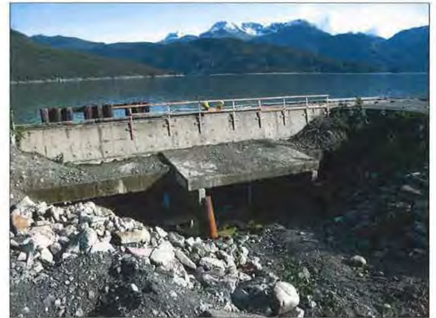
3 38 CELL 4 - CONCRETE CAP & SHORING
